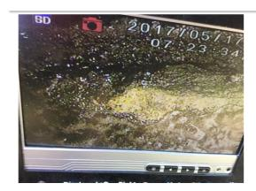
"Several of the mortar joints have crumbled from expansion of the flue tiles due to the chimney fire"
